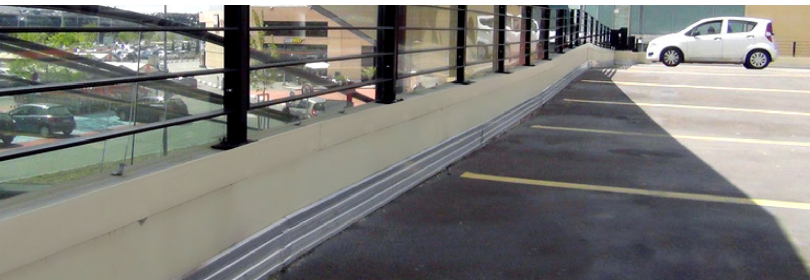
Solinet® Bridge ans parking
